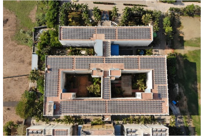
Solar Panels 300 kVA Installed
