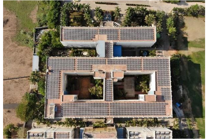
Solar Panels 300 kVA Installed
